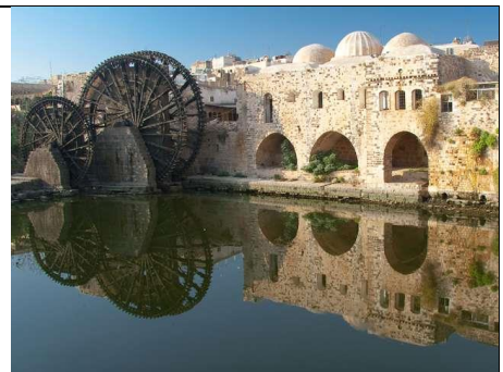
Double water wheel used to irrigate gardens in the country of Syria
